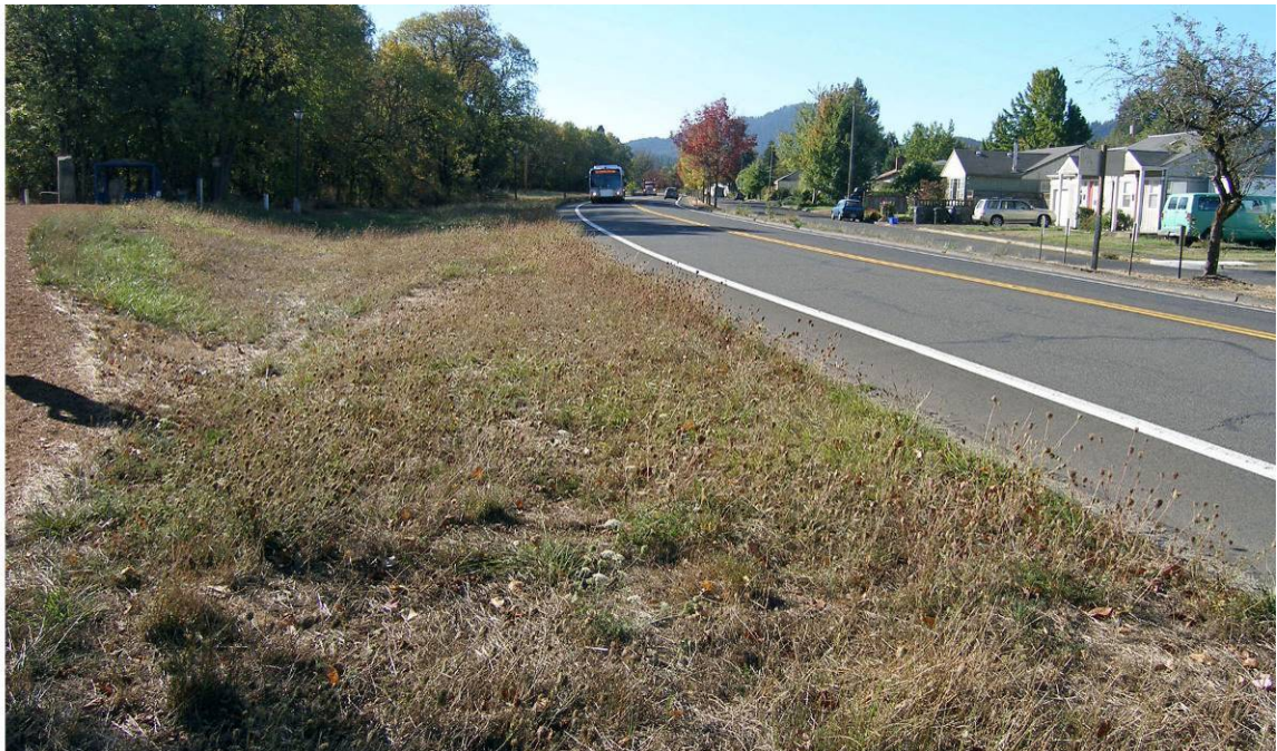
Figure 6.1-2. Raised Roadbed and Drainage Swale East of Amazon Parkway
