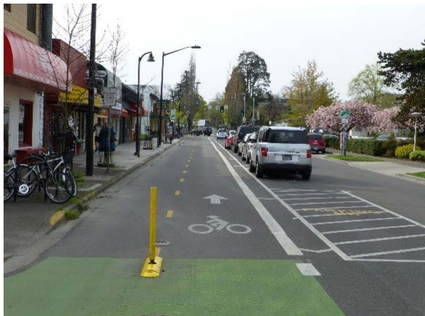
Cycletracks are on-street bicycle facilities separated from vehicle traffic. Cycletracks can be one-way or two-way bicycle facilities.
