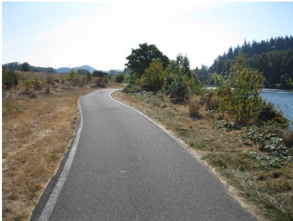
A shared-use path is separated from road traffic and may be used by both pedestrians and cyclists.
