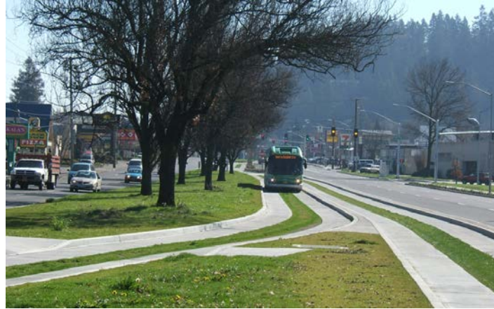
Dedicated transit lanes are separated from traffic and may only be used by buses.
