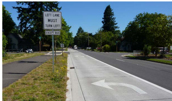
Business access and transit (BAT) lanes are lanes used by buses, but may also be used by right or left turning traffic.
