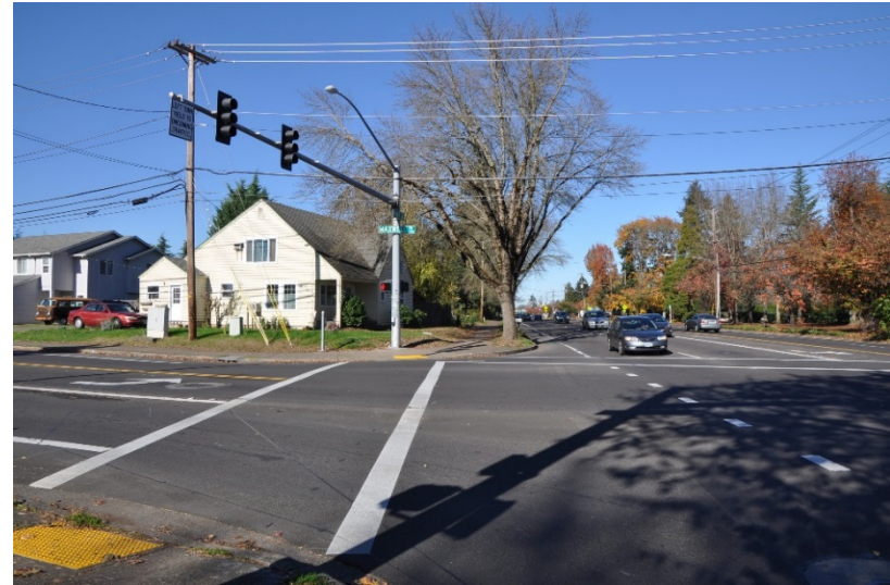
Photo 23. West side of River Road, at Maxwell Road, looking north
