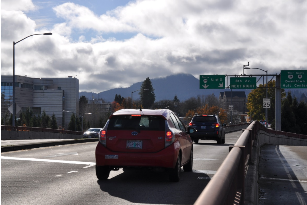
Figure 3.1-1. Coburg Road/Mill Street at East 6th Avenue Looking South (Spencer Butte in Distance)
