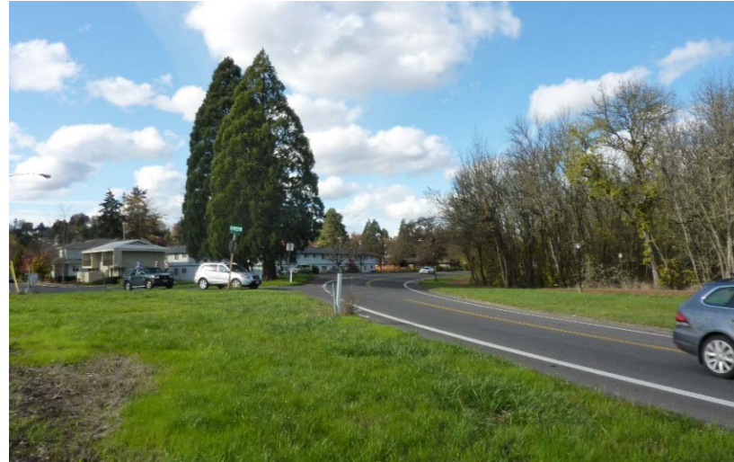
Photo 43. Amazon Parkway, at East 27th Avenue, looking northwest
