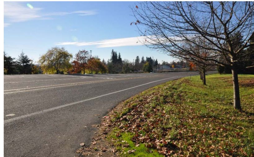
Photo 25. West side of River Road, at NW Expressway, looking west
