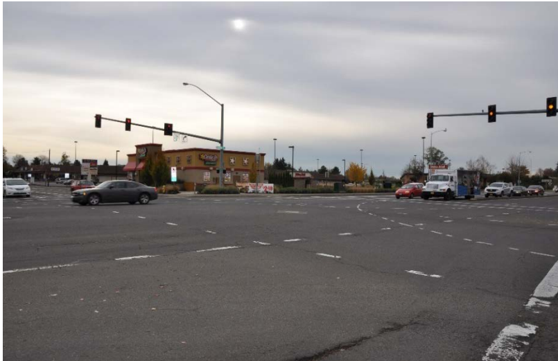
Photo 1. North side of Barger Road, at Cubit Street, looking southwest
