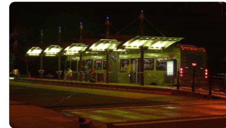
Bus stop lighting at an EmX station
